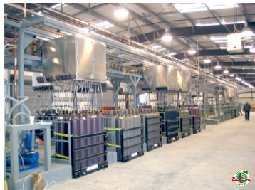
Fully Automated Cylinder Filling Station
